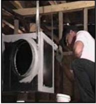
One of the cheapest and most effective ways to reduce heating loss in your home is to seal leaky ductwork. Over 20% of the average home's heating and cooling bills go to duct leakage in attics or crawlspaces. Sealing your ducts with mastic (a paste-like substance available at most home improvement stores) can substantially decrease the amount of conditioned air being wasted. A homeowner can spend as little as \$10 and a few hours of time to accomplish this task.
