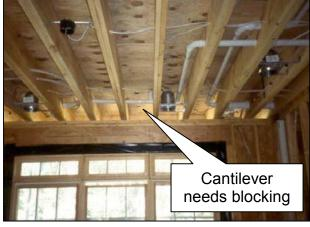
The truss company will design an upright solid piece of wood at the point where blocking is needed if specified during the design phase.
