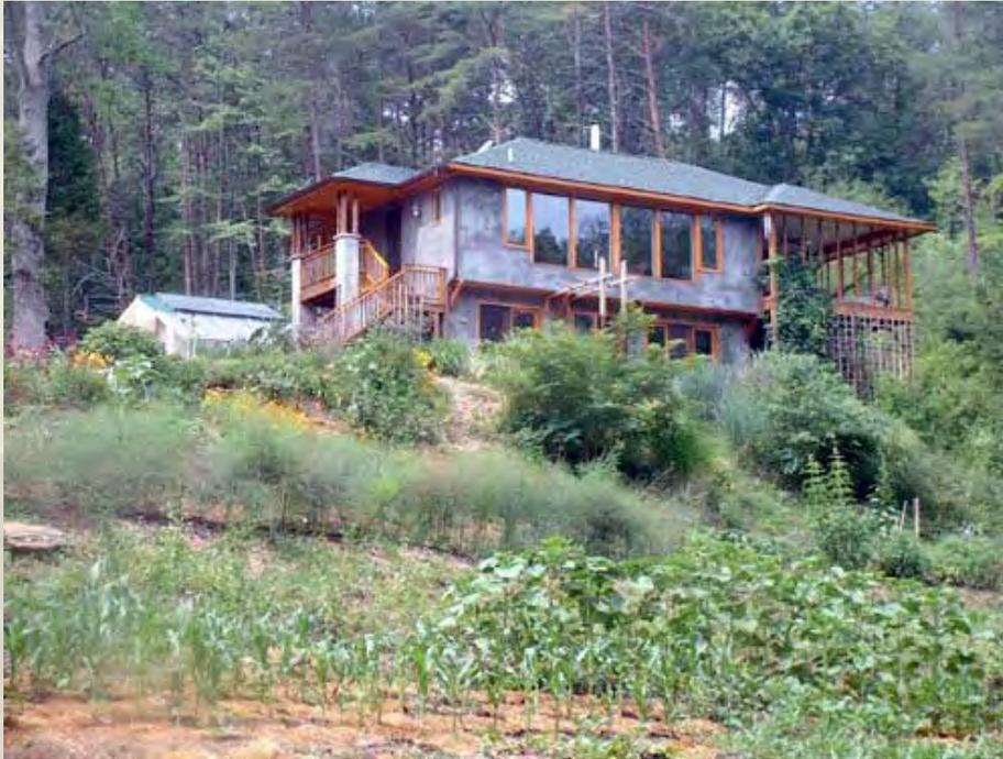
The Cady-Guyton Home is built into a south facing hill that allows for a passive solar design with an earth-bermed first floor (daylight basement). There is a woodshop (20x30ft) and a small solar greenhouse in addition to the 1550 sq ft. living space.
