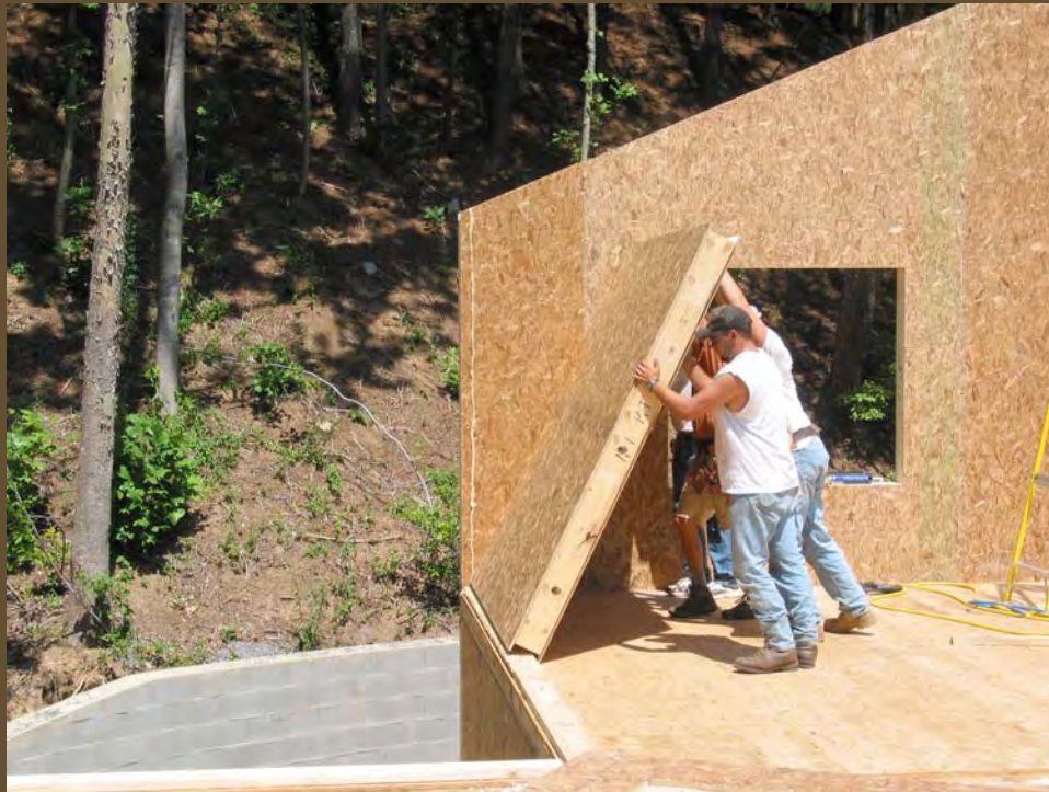
Setting up SIPS walls
