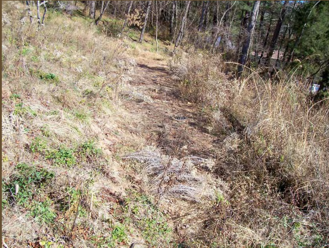
The bio-retention trench that captures runoff from the building & filters it before draining into the Swannanoa River.
