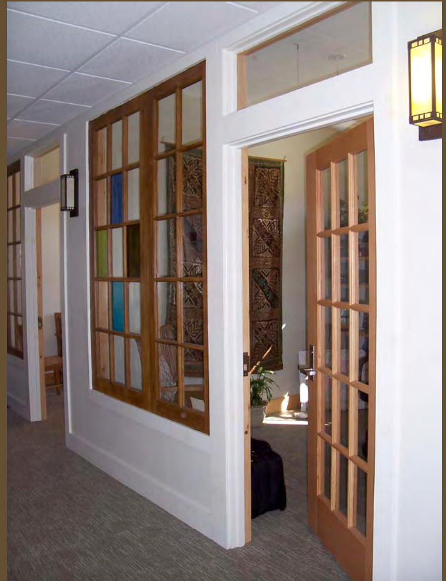
Salvaged doors with stained glass allows day lighting to enter most of building, local recycled carpet, and low VOC paint.
