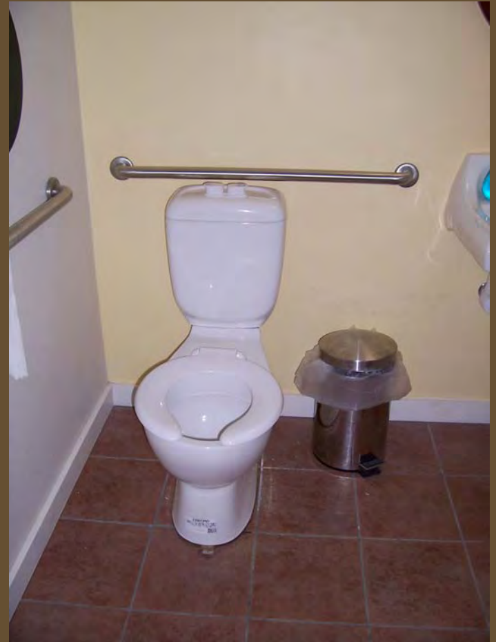
Dual-flush toilet and high recycled content tile in lower level restroom.
