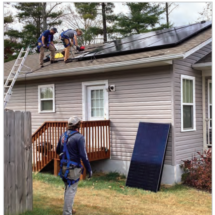
Sugar Hollow team installs panels for a recipient in Arden.
