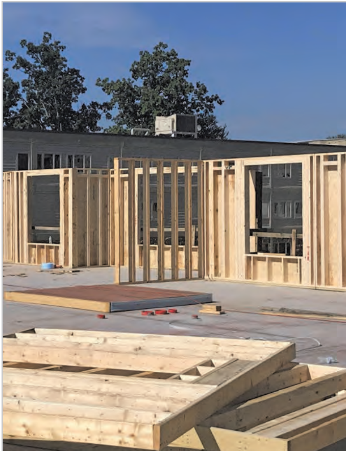
Installing panelized wall systems. CHRISTINE DAVIS PHOTO
