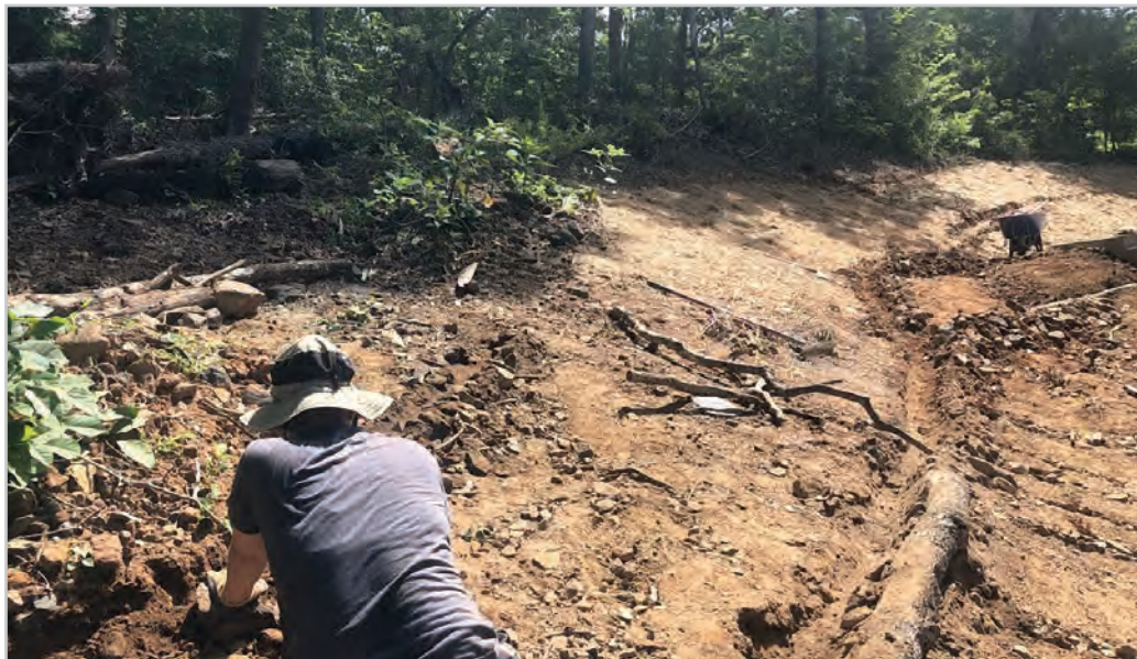
Examples of steep slopes harmed by excavation, in a state of unstable dynamics. Field staff conducting “emergency services,” to stabilize the slope, using stones and logs on site to contour, slow, and infiltrate water across the bare slope, instead of the water coursing down, taking the sediment and mountain with it. KERI EVJY PHOTOS
