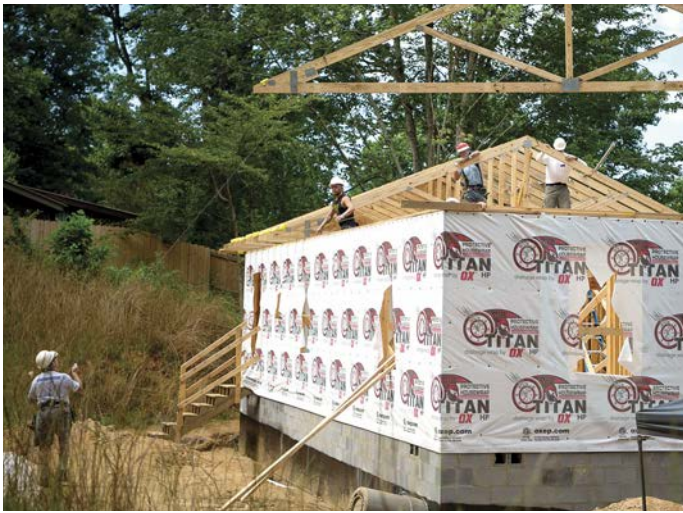
Asheville Habitat staff and volunteers install roof trusses at the jobsite in Mars Hill. The construction of this home was completed in December of last year. ASHEVILLE AREA HABITAT FOR HUMANITY PHOTO
