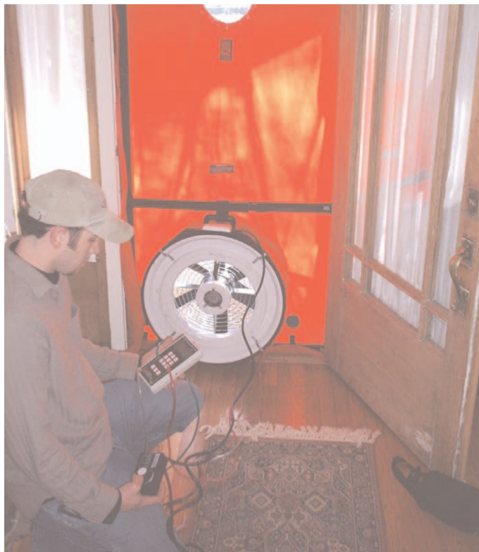
Setting up a blower-door test.
