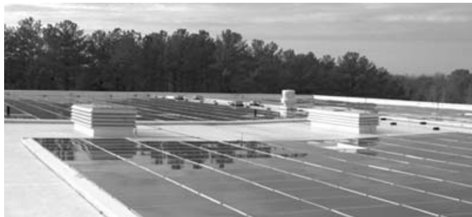
The EPA’s National Computer Center has a 100-kilowatt (photovoltaic) solar roof, the largest in the Eastern U.S.
