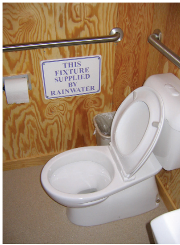
Prairie Ridge Eco-Station in Raleigh uses rainwater to flush classroom toilets. This enriches student curriculum and promotes water conservation.
