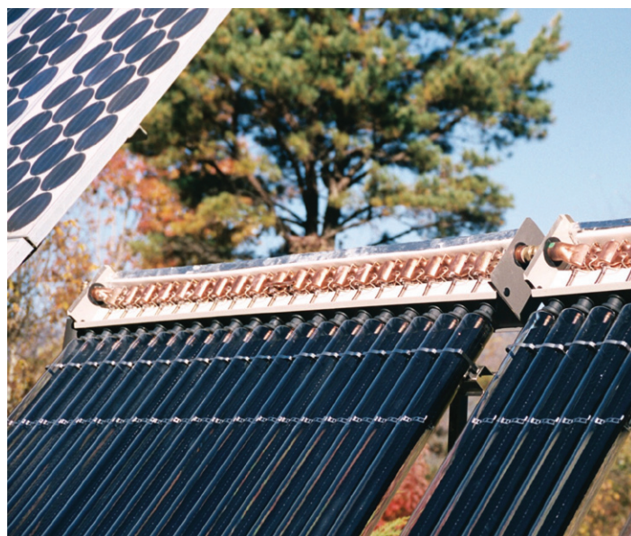
An array of solar evacuated tube collectors, showing how they connect to the manifold at the top.
