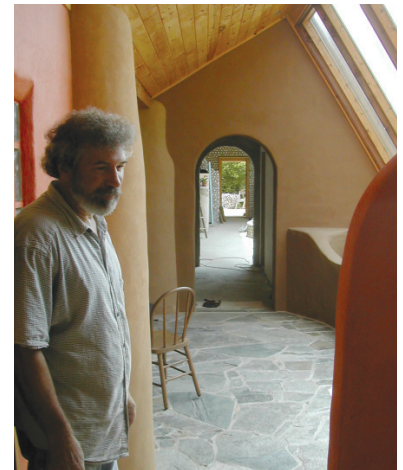
The Earthship's sloped glass design allows for optimal collection of winter sunlight, and keeps the interior relatively cool in the summer months when the sun is higher in the sky.
