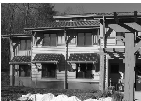
Awnings above south facing windows of the EcoDorm are equipped with solar panels. Outside, permaculture techniques are used to create an "edible landscape" (photo by Rebecca Bowe).
