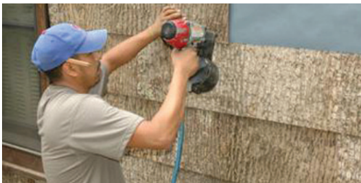
Applying bark house shingles (photo by Todd Bush).
