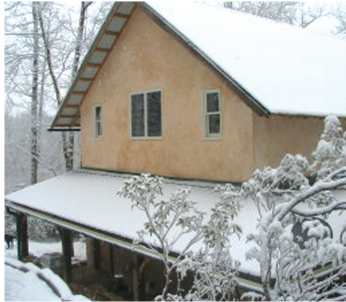
Withstanding the elements of the Appalachian Mountains is no problem for this straw bale home (photo by Bobby McHugh).
