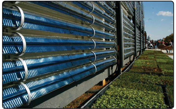
Solar evacuated tubes at the University of Cincinnati team house at a Solar Decathlon event in Washington, D.C., in October 2007.
