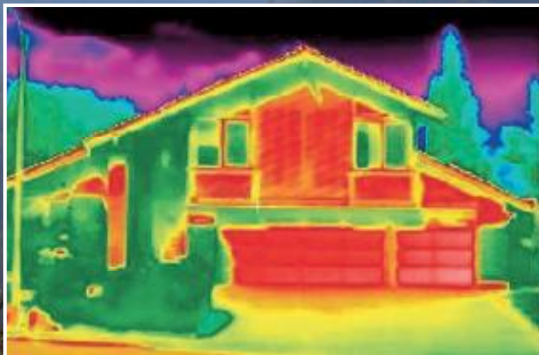
Infrared Photo - Energy Loss - Poor Quality Construction
