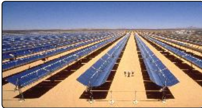
Nevada One, a utility-scale concentrating solar power plant in Boulder City, Nevada. photos courtesy of SEIA
