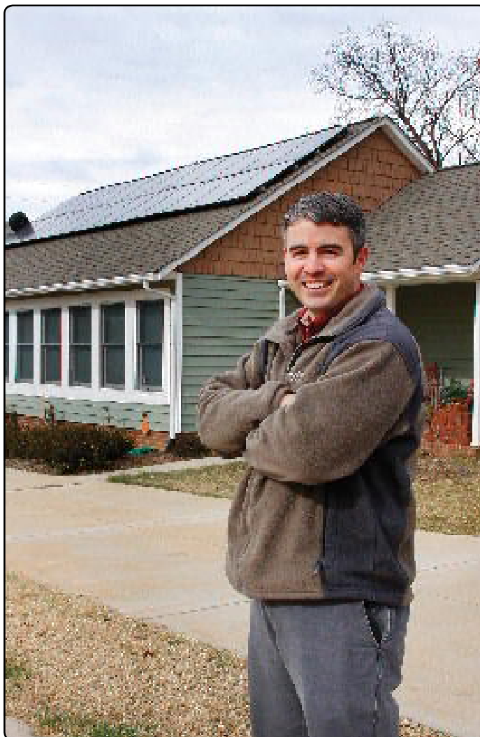
Rob Howard, construction project manager for Catawba Valley Habitat for Humanity, oversaw the construction of this zero-energy home in Hickory. photo by Jonathan Welch
