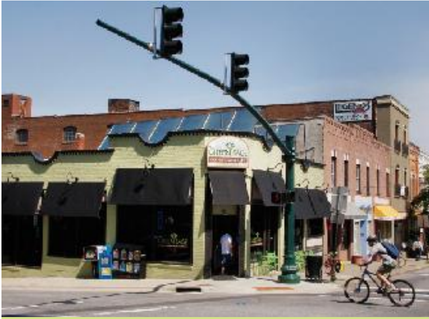
Look on the sunny side: The rooftop solar panels at Green Sage Coffeehouse & Café power the restaurant's hot-water system. photos by Jonathan Welch
