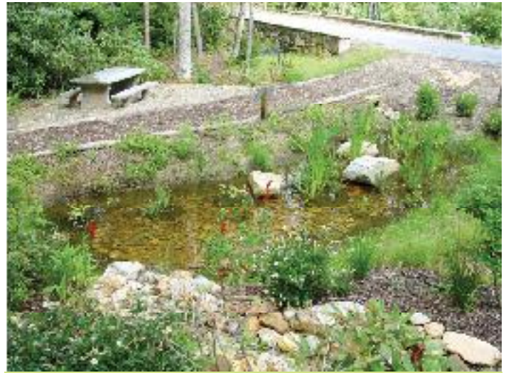
Constructed wetland at Drover's Road Preserve in Fairview: This decorative pond shows that stormwater can produce aesthetically pleasing results, in addition to preventing erosion and filtering pollutants. photo courtesy of Equinox Environmental
