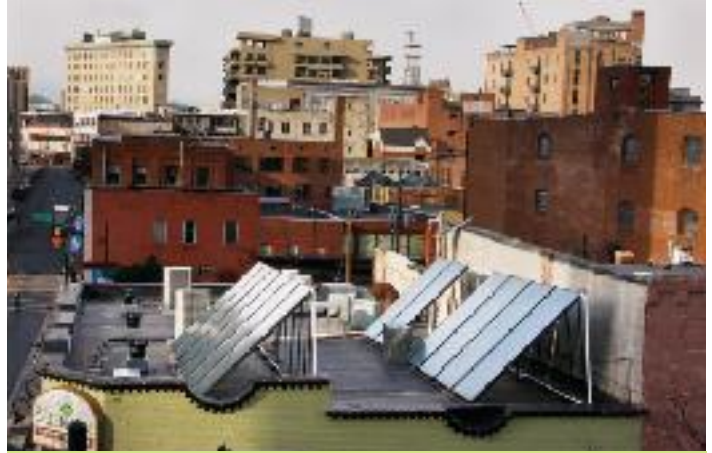
The changing skyline: Green Sage owner Richard Talley hopes these solar panels will entice others to try the technology.
