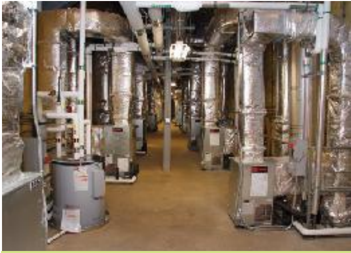
The geothermal nexus: The Cherokee Central School campus is heated and cooled by a geothermal system that draws on the earth-power of about 300 wells. photo by Jonathan Welch
