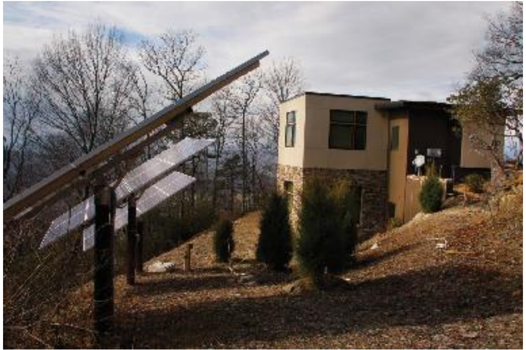
Solar tilt: Yves Naar's mountaintop perch uses a combination of approaches to achieve net-zero-energy use, including the system powered by these solar panels. photos by Jonathan Welch
