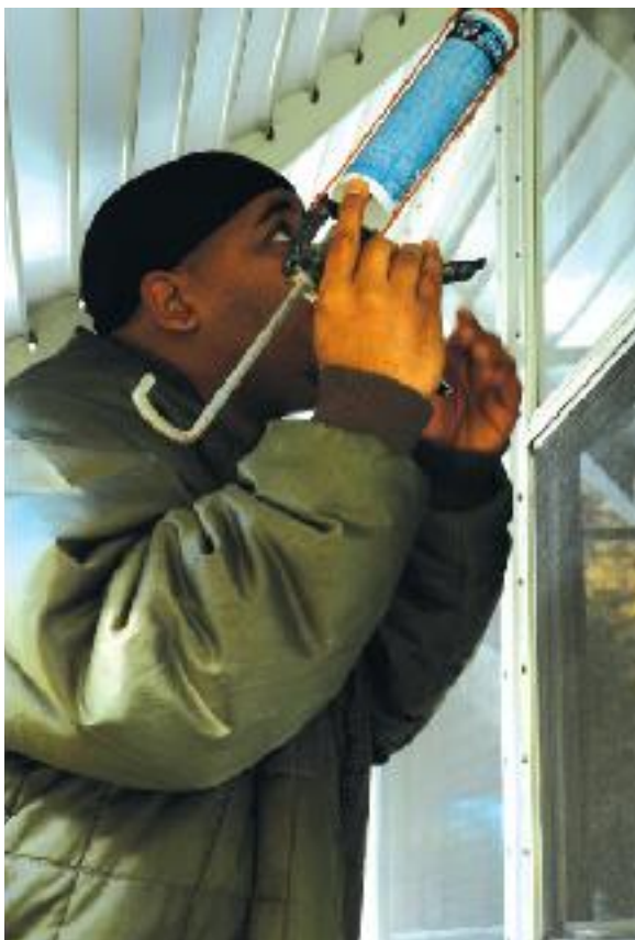
Low-cost efficiency method: Caulking and weather stripping are two of the least expensive approaches for improving energy efficiency as demonstrated by Delario Cato. photo courtesy of Asheville GO!
