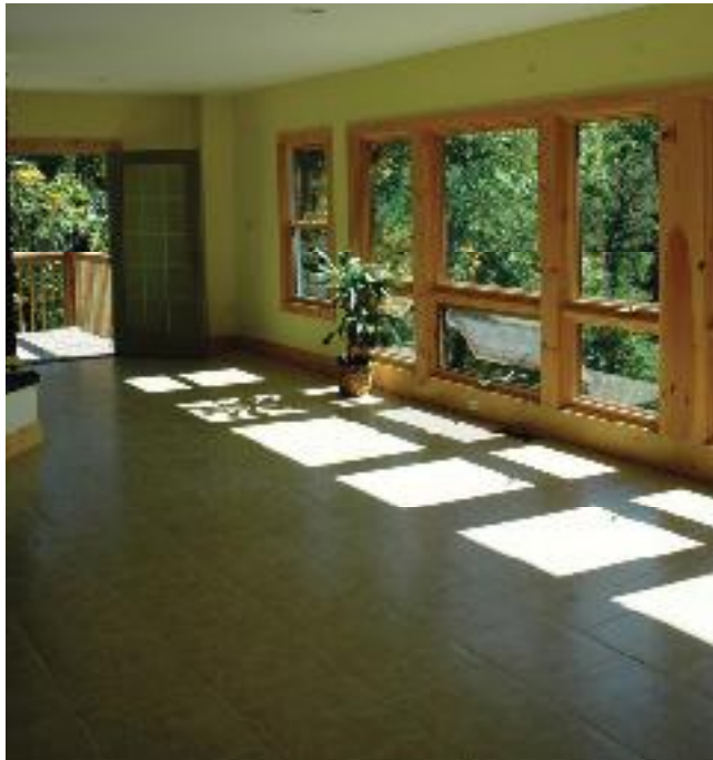
No-fuss solar: Using passive-solar design, including a calculated amount of thermal mass and glazing, can supply significant amounts of the heating needs for the home, as at Brian Knight's Montford home. photo courtesy of Candice Black
