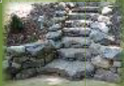
Traditional Stonework chimneys, retaining walls, patios and more.
