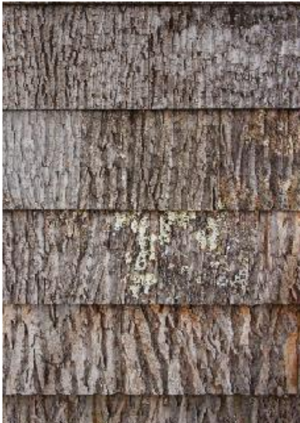
Bark on the side: One oft-discarded byproduct of the milling process is bark, used here as siding on a net-zero-energy house.
