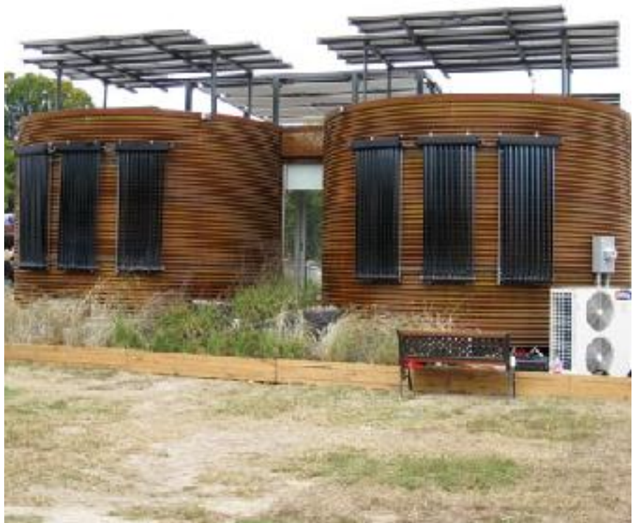
Look of the future? Every home at the Solar Decathlon used solar-thermal water-heating systems, and all featured their own unique look.
