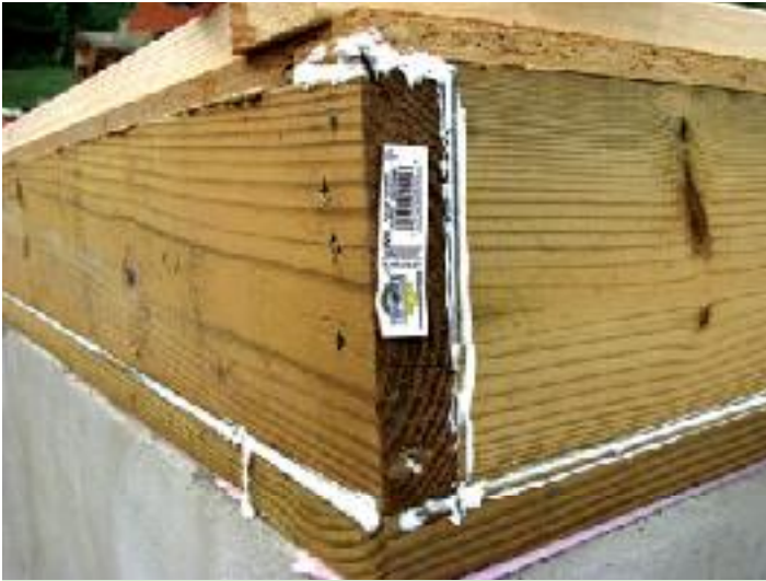
Seal it: Air sealing is essential to an energy-efficient home.
