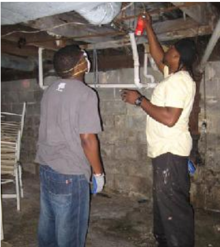
GO green: Green Opportunities members work on air and duct-sealing techniques, which save energy and cut utility bills for low-income homeowners.
