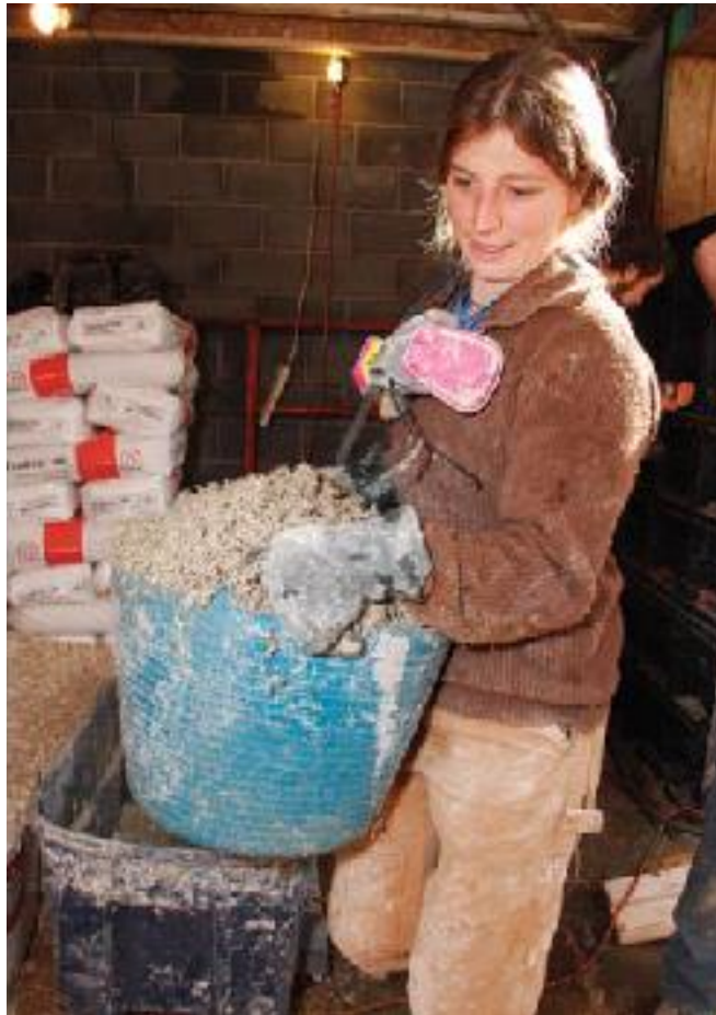
Strong stuff: Hempcrete walls have good insulating properties and are vapor permeable — the material can absorb or shed water in response to changing humidity levels in the home.
