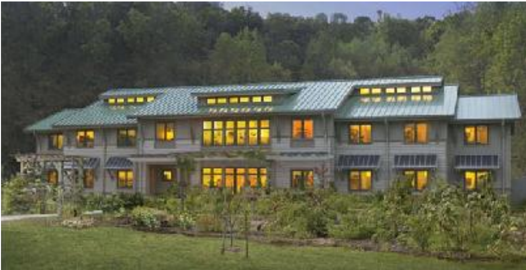
Aligned to the sun: Warren Wilson College's eco dorm, shown here at twilight, utilizes several passive solar techniques.
