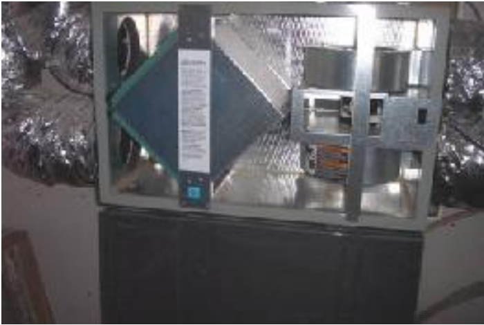
Fresh system: An Energy Recovery Ventilator is an efficient way to provide fresh, prefiltered air throughout the home.
