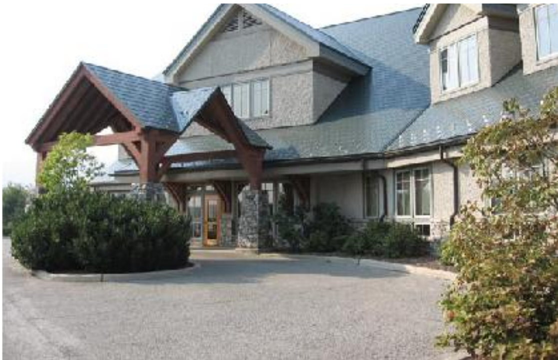
Beneficial surface: This pervious concrete parking surface at Western Carolina Retinal improves safety, reduces runoff and is a cost-efficient approach to treating water quality.
