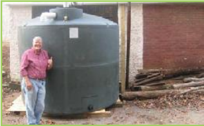
Size: 2,000-gallon above-ground system Use of water: Used as landscape irrigation for gardens Where: Calvin Allen & Maria Fire Residence, Asheville, N.C. System installed by: Cistern Sister photo by Kathryn Cartledge Allen
