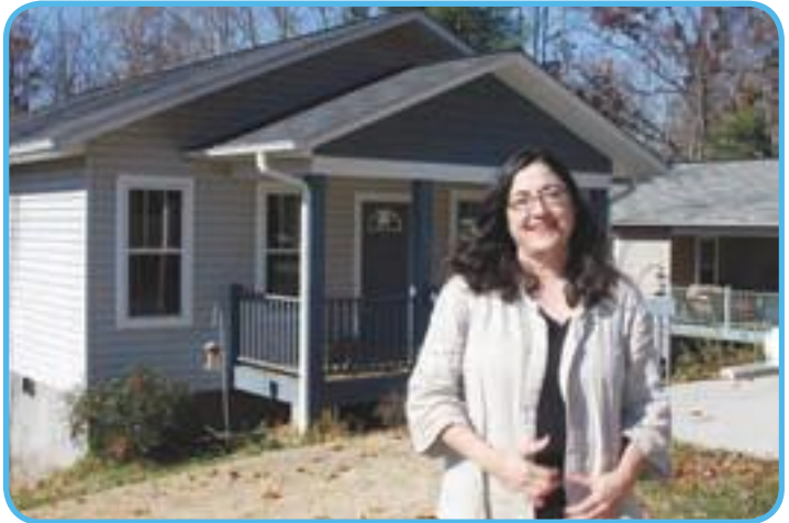
Happily relocated: Elaine Sargent settled her family into this NC HealthyBuilt, ENERGY STAR-certified home in Enka Hills after moving from New Orleans in the wake of Hurricane Katrina.
