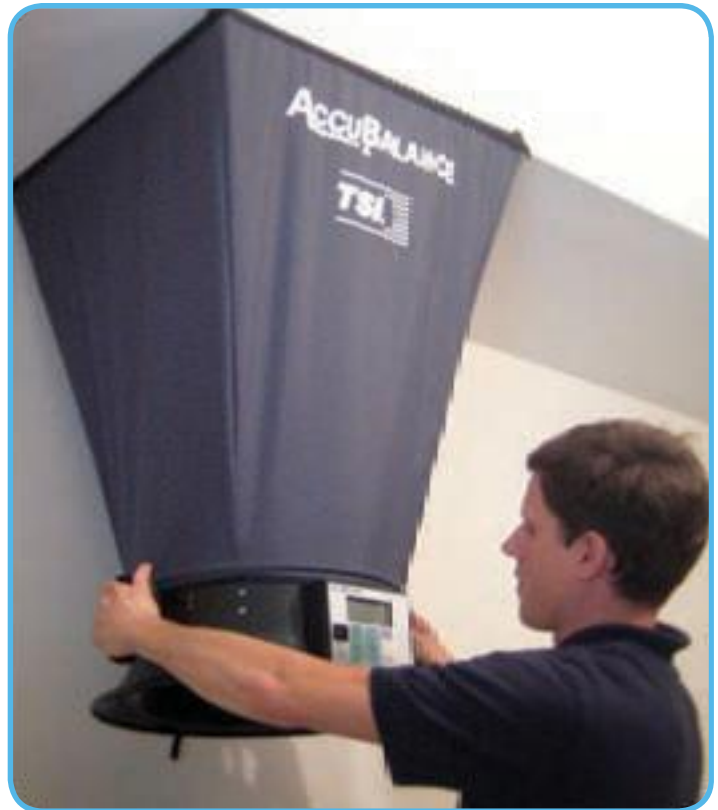
A new requirement: Under ENERGY STAR Version 3.0, a diagnostic test ensures the HVAC system is providing adequate airflow at each room to keep the home comfortable and operating efficiently. photo courtesy of Home Energy Partners
