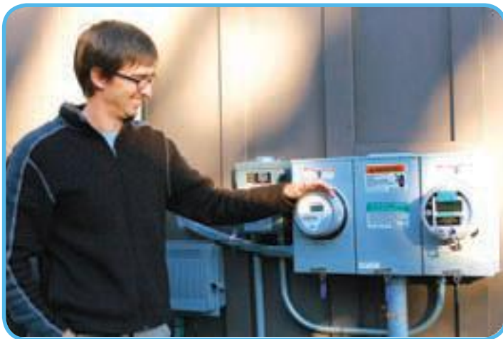
Selling solar power: This dual metering system lets homeowner Ben Edson see both how much solar-generated electricity his home uses and how much of this electricity he and his wife are selling back to Progress Energy at a rate of 24 cents per kilowatt hour.
