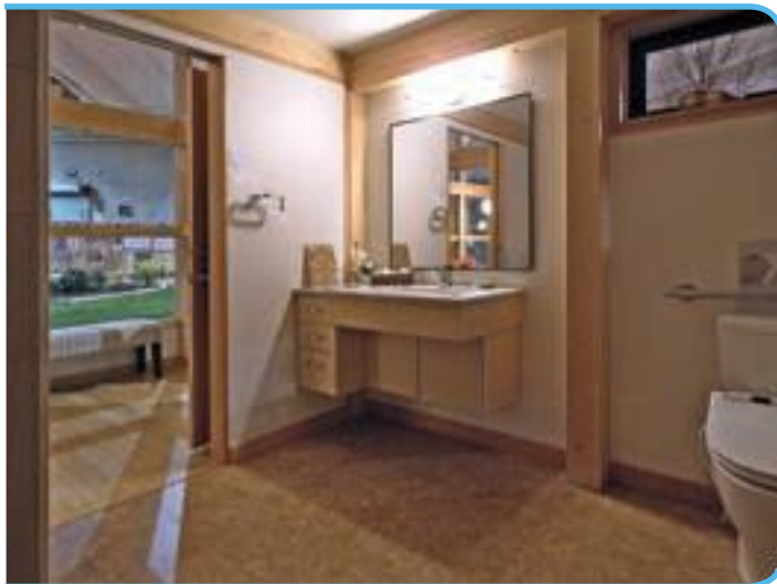
Open space: This bathroom sink allows a wheelchair-bound resident to roll up to the vanity. photos by Dale Lang
