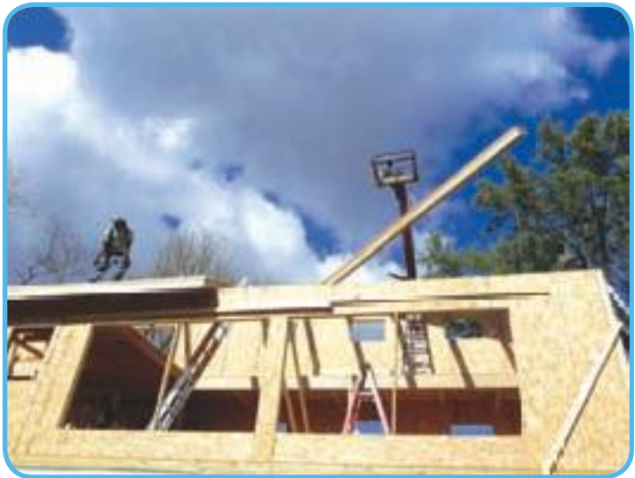
Well insulated: SIPs are one way to achieve maximum insulation in a wall and decrease thermal bridging. photos by Matt Siegel
