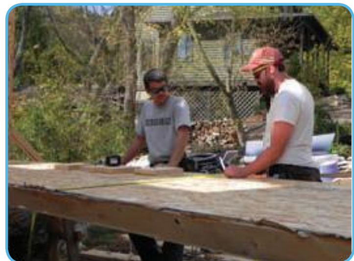
A SIP at a time: Structural insulated panels are composed of foam insulation sandwiched between a "skin" of oriented strand board — the combination creates both a strong wall section and a continuous layer of insulation.
