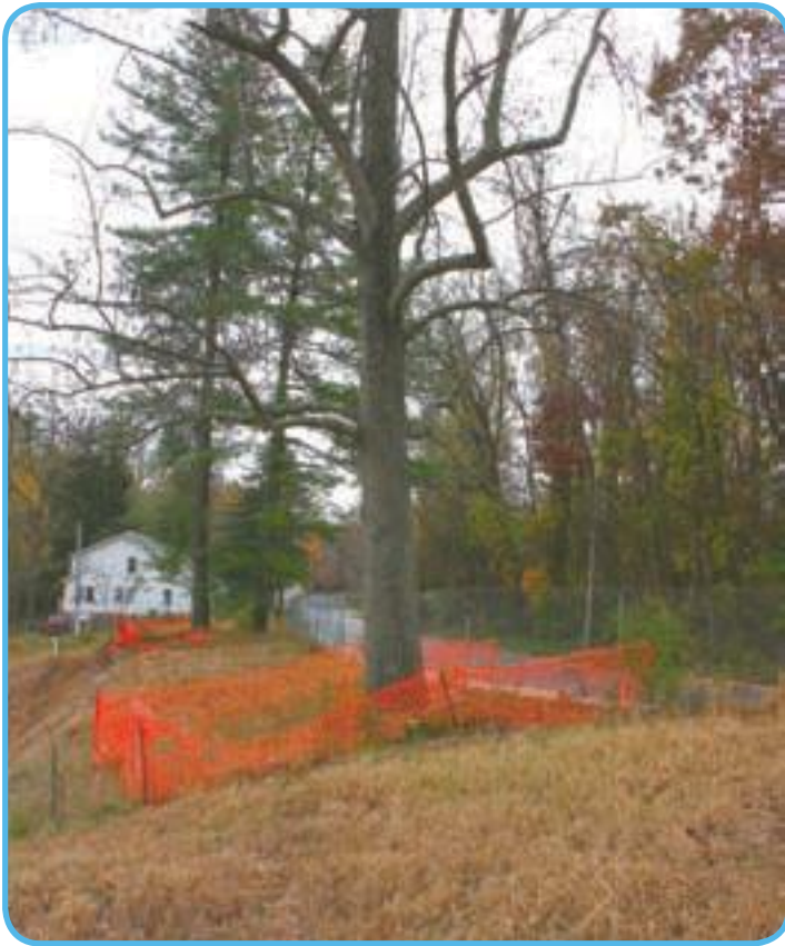
The zone: The most effective way to protect a tree during construction is to create a tree-protection zone.
