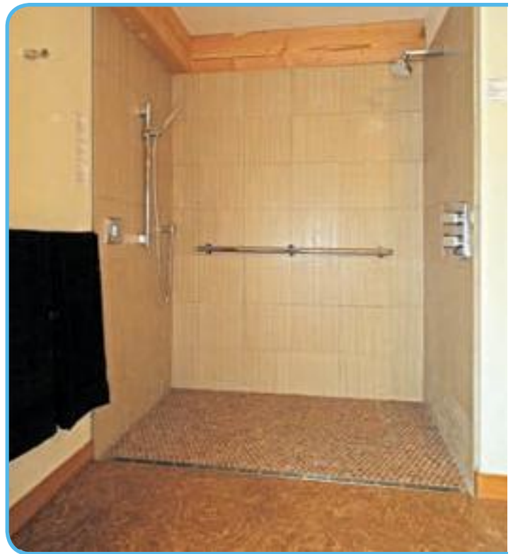
Accessibility: A sill-less shower is level with the floor for easy entry and adds drainage to the bathroom.
