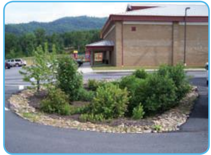
School lessons: Bethel Elementary School in Bethel, N.C., uses a Best Management Practice for collecting stormwater runoff from the school's roof and paved surfaces so it can slowly seep back into the ground. photo courtesy of Equinox Environmental
