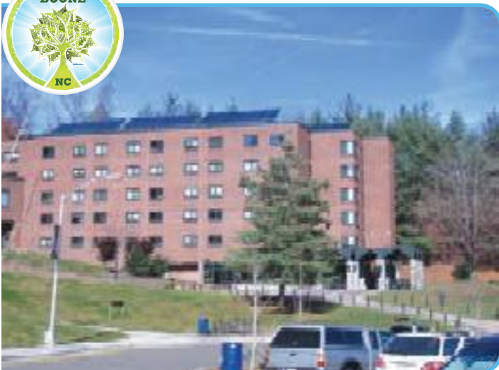
Something old, something new: These are not the same dorm rooms of yesteryear. While the structure for the dormitory, Frank Hall, was built in the 1970s, a slew of new green features earned it a Gold LEED certification.
