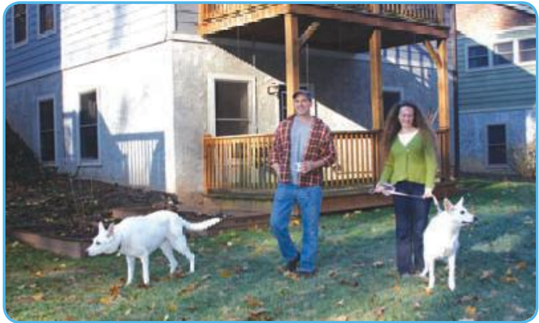
Happy, green and bermed: In WNC, we call it a walk-out basement; Amy Musser and Matthew Vande say the house is bermed — being built into the hillside (and having a geothermal system) uses the earth's relatively constant temperature to heat and cool the house.
