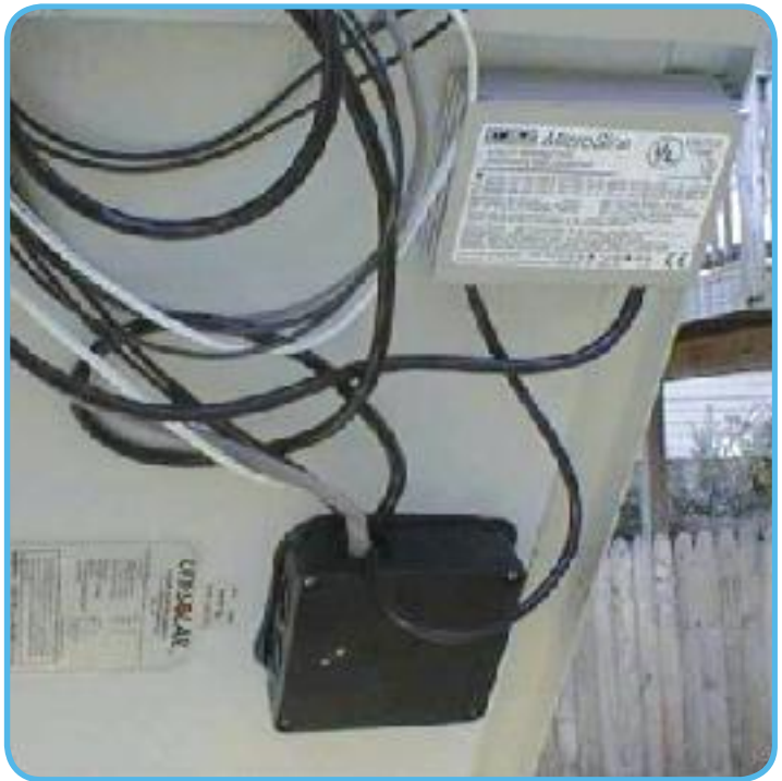
Just a little black box: One of the most innovative changes in the solar industry is the micro-inverter, which can — among several functions — report on the output or any malfunctions in its panel individually. photo courtesy of Johns Hopkins physics department
