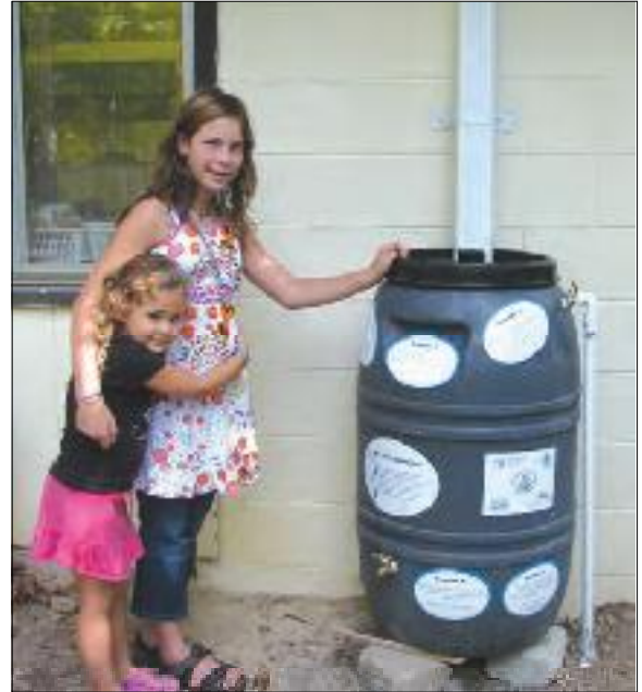
"R" is for rain barrels: The Reading, Riding and Retrofit program helps schools become more sustainable, by adding such features as a rain barrel.
