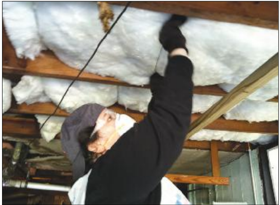
Out with the old: Held in place by little more than lengths of wire, most older fiberglass insulation sags over time. Spray-foam insulation is more effective — but can be more expensive.
