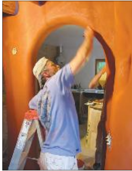
The personal touch: Steve Kemble burnished homemade clay-based plaster in this archway.
