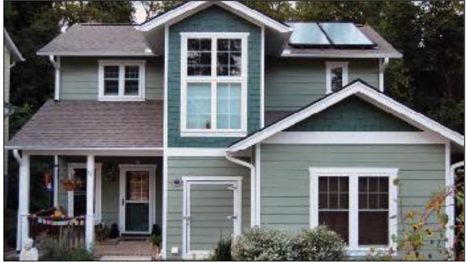
Earth friendly: In West Asheville, the Gaia community features NC HealthyBuilt Homes like this one, done in the locally common Arts and Crafts style — with solar.
