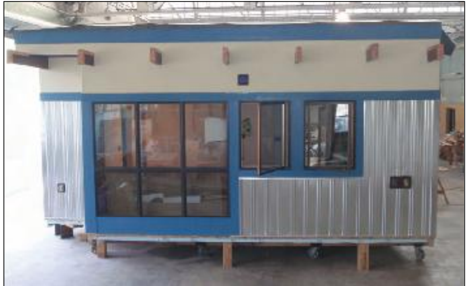
The little house that could: The smallest known LEED home packs an impressive array of environmentally friendly features in its 280 square feet of space.
