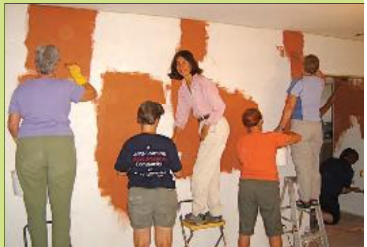
Hands-on training: People work the lumps out of native clay; students apply homemade clay-based paint over latex during a workshop.
