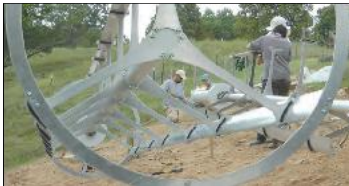
Space saver: Not all wind turbines feature large propeller blades. These vertical-axis turbines are quiet and bird-friendly.
