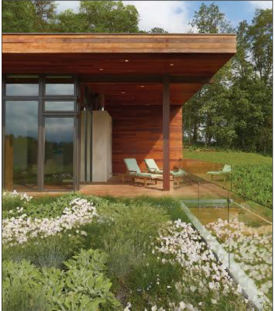
Coming together: A green roof seamlessly integrates the living spaces of this home with the surrounding landscape.
