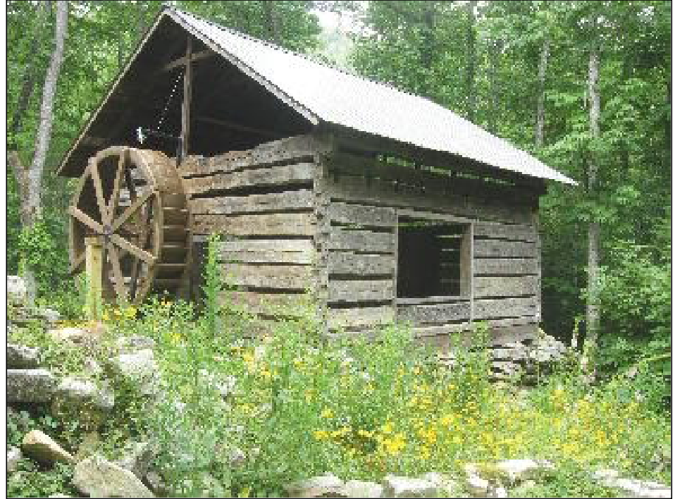
Grist mill reborn: Logs from an 1840s Piedmont cabin became Hickory Nut Forest's new mill, built next to the foundation of an old gristmill on the property.
