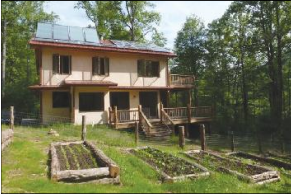
Community: This passive- and active-solar home illustrates how each member of the community contributes to the zero-energy goal.
