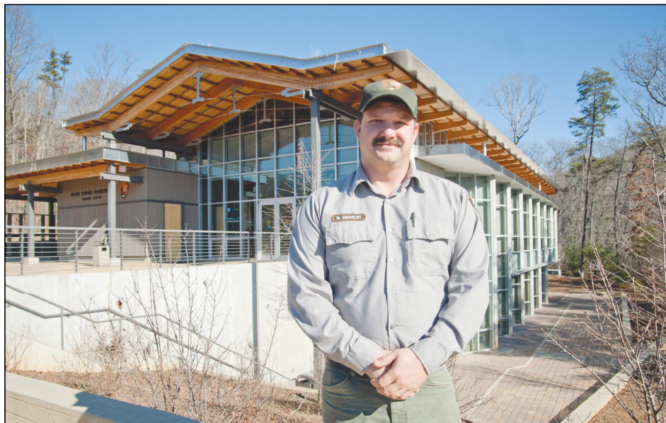
Trial and error: After five years maintaining the LEED-certified Blue Ridge Parkway Visitor Center, staff have learned through trial and error which green features are working best and which need adjustment, says Brandon Hensley, National Park Service maintenance mechanic.
