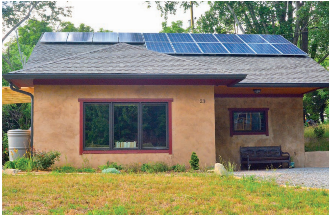
Located on Trade Street in the River Arts District of Asheville, this home was built by Cady & Guyton Construction. The structure features solar panels, rainwater collection and a high-efficiency water pump. Garret K. Woodward photos
