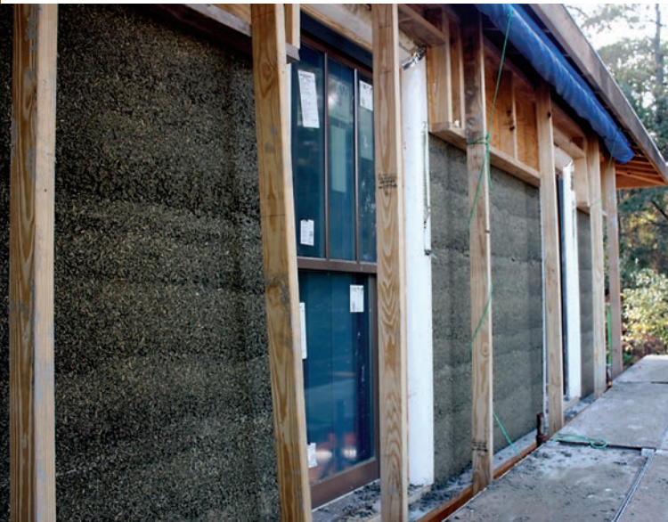
Hempcrete installation. Alembic Studio, LLC photo
