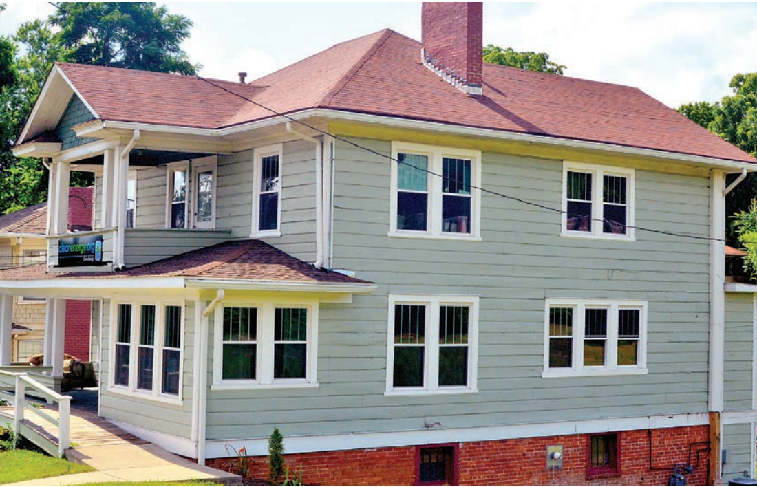
The Southern Alliance for Clean Energy in downtown Asheville. Basement encapsulation to reduce moisture in the SACE office. (below) Garret K. Woodward photos
