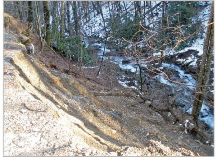
Left: Long Branch natural debris flow, Maggie Valley, Jan. 15-16, 2013. Above: Road embankment failure/debris flow, Maggie Valley, Jan. 15-16, 2013. Photos by Appalachian Landslide Consultants, PLLC
