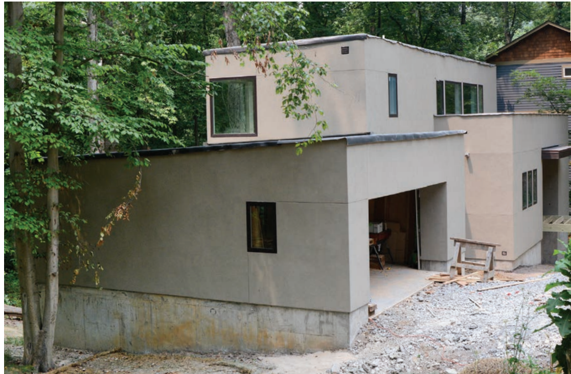
Located near Biltmore Village, this residential home utilizes green materials, with the key to the structure being structural insulated panels (SIPs). Bob Callahan (below). Garret K. Woodward photos
