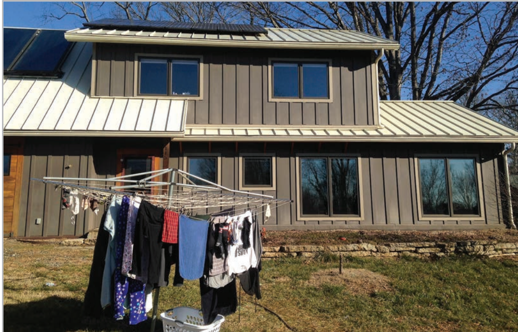
The photo above shows a home using four forms of solar: solar PV, solar hot water, passive solar, and solar clothes drying. Passive solar design is popular with net-zero energy home builders. It's definitely not a requirement, but since these homes have to be oriented for South-facing roofs anyway, it can capture that free heating energy from the sun. Amy Musser photo
