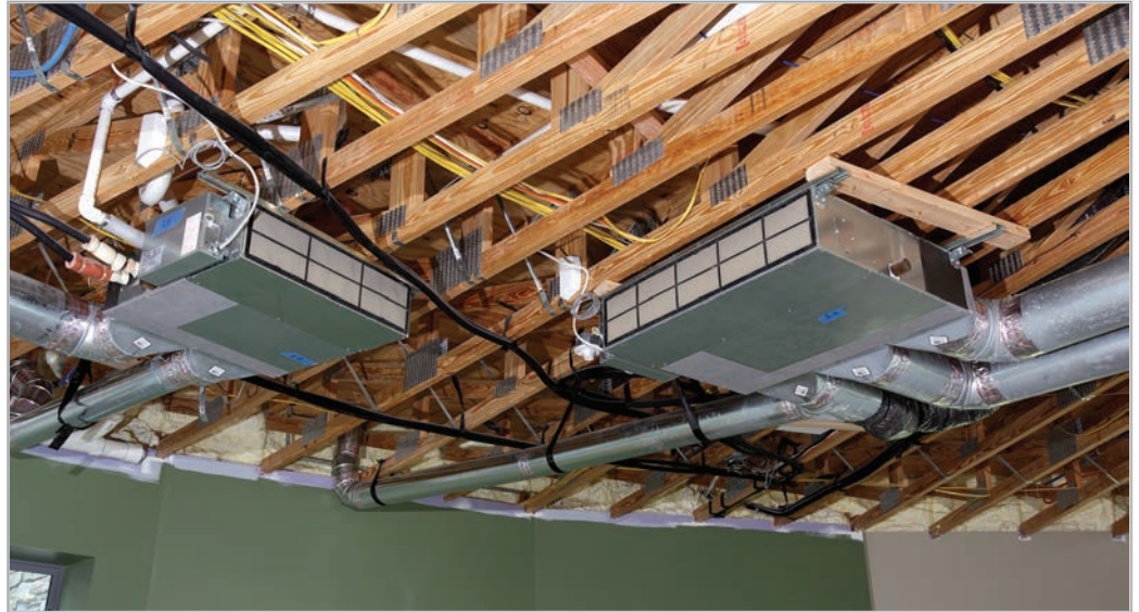
(Above) Two "horizontal-ducted" mini-split air handlers fit nicely in the ceiling of a basement and serve two halves of this large super-insulated house (<4,000 square feet) in State College, PA. (Right) Mini-split outdoor compressors look a little different than traditional heat pump compressors too, and they're generally much quieter. LEIGHA DICKENS PHOTOS
