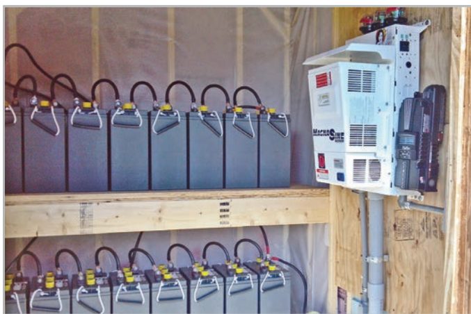
(Above) Roof-mounted solar photovoltaic panels offer clean energy while saving space in your yard. For best output in most cases, solar PV panels should be within 20 degrees of true south. (Left) Battery banks are integral to off-grid systems, yet do not need much floor space. This 48-volt battery bank provides power to the adjacent inverter which produces conventional 120 volt AC for the home. SUNDANCE POWER SYSTEMS PHOTOS
