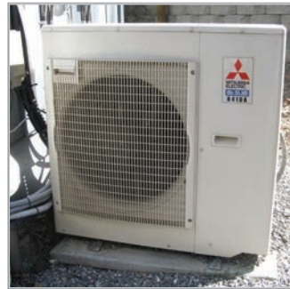
(Above) Two "horizontal-ducted" mini-split air handlers fit nicely in the ceiling of a basement and serve two halves of this large super-insulated house (<4,000 square feet) in State College, PA. (Right) Mini-split outdoor compressors look a little different than traditional heat pump compressors too, and they're generally much quieter. LEIGHA DICKENS PHOTOS
