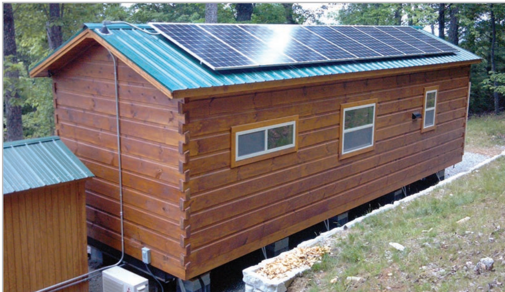
(Above) Roof-mounted solar photovoltaic panels offer clean energy while saving space in your yard. For best output in most cases, solar PV panels should be within 20 degrees of true south. (Left) Battery banks are integral to off-grid systems, yet do not need much floor space. This 48-volt battery bank provides power to the adjacent inverter which produces conventional 120 volt AC for the home. SUNDANCE POWER SYSTEMS PHOTOS
