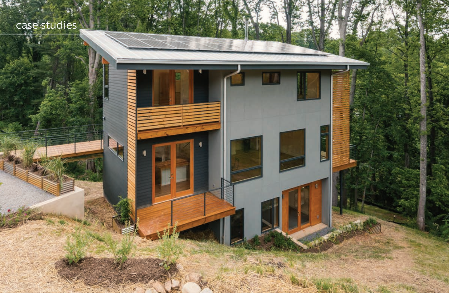
The first home is nearly complete in the new Shelburne Woods subdivision, where each home will meet Green Built Homes Platinum, Net-Zero Certification.
