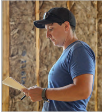
Jessica Arrowood of Vandemusser Design reviews a Green Built Homes checklist during a framing and insulation inspection of a house under construction in The Villages at Crest Mountain in Asheville. DAYNA REGGERO PHOTO
