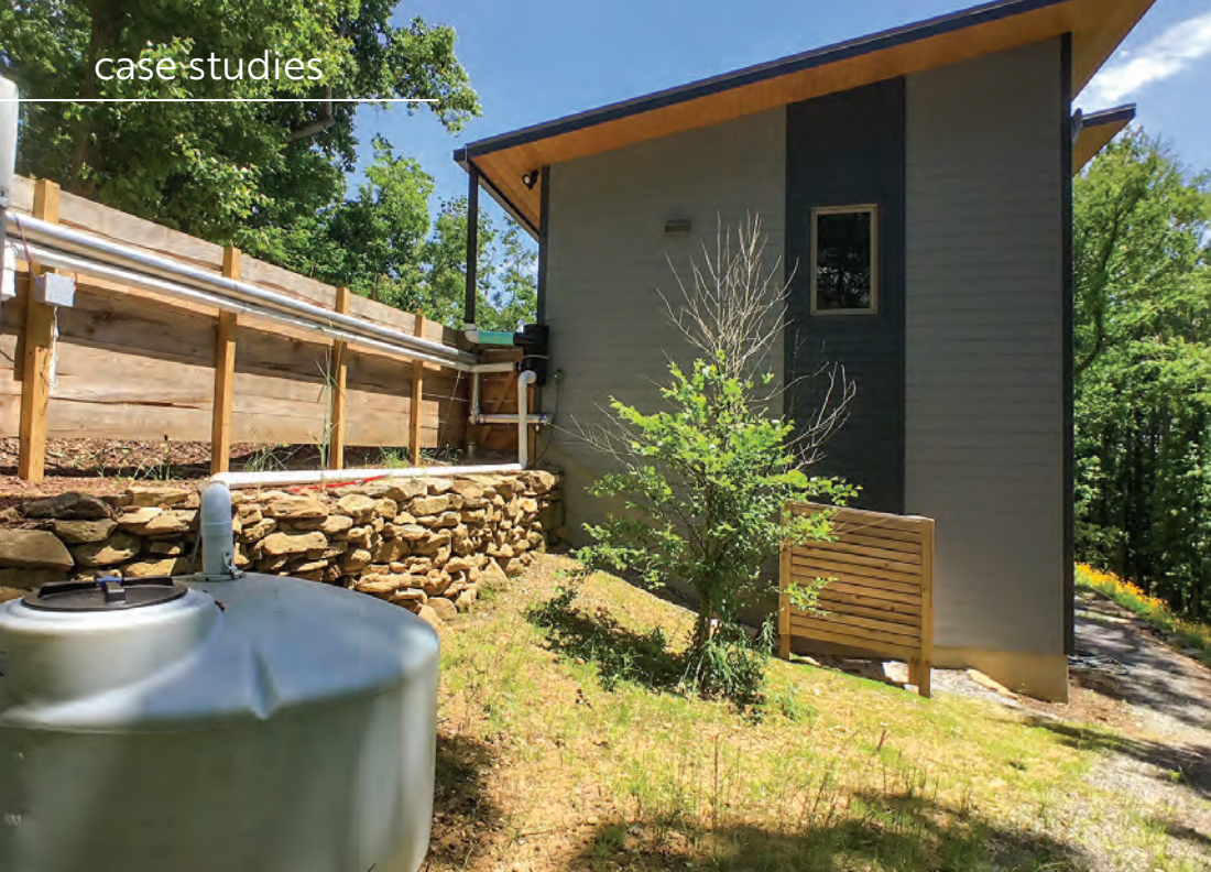
This Swannanoa home received a Green Built Homes Gold certification, in part due to the rainwater collection system installed by the project team. EVERGREEN CONSTRUCT PHOTOS
