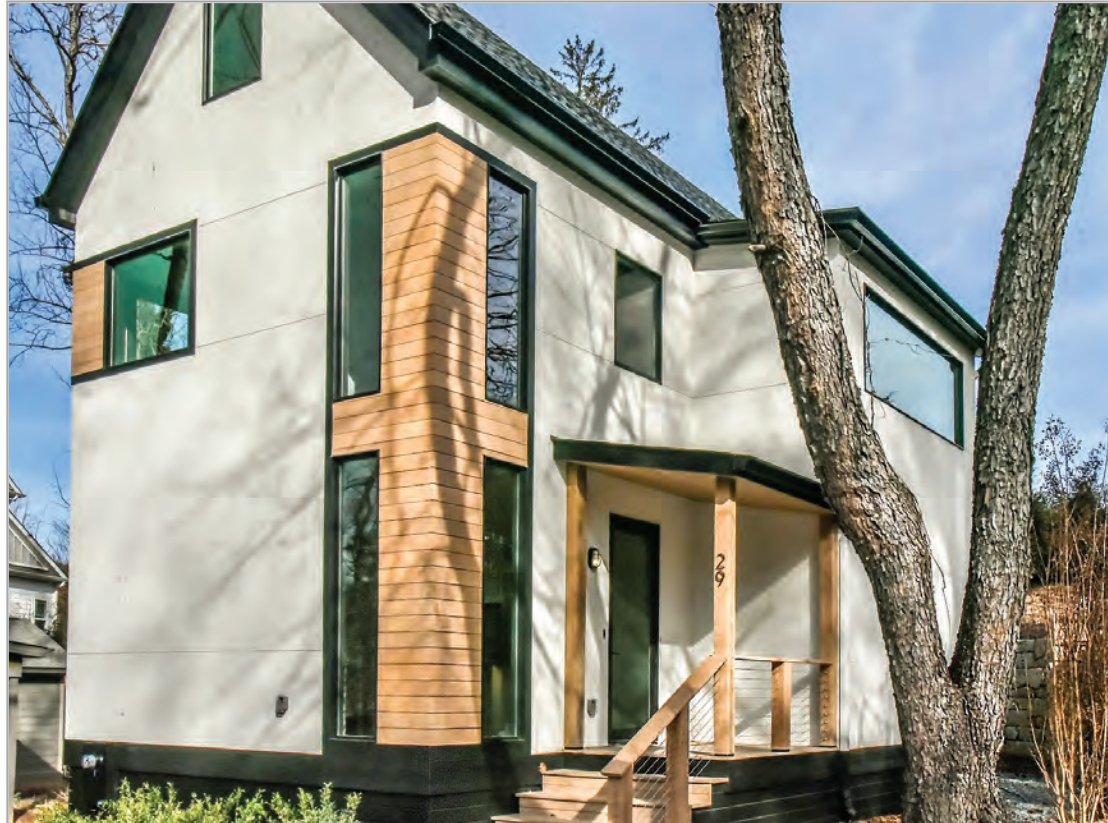
This Asheville home was designed to serve as a prototype for high-performance homes. TRILLIUM PROPERTIES OF ASHEVILLE PHOTOS
