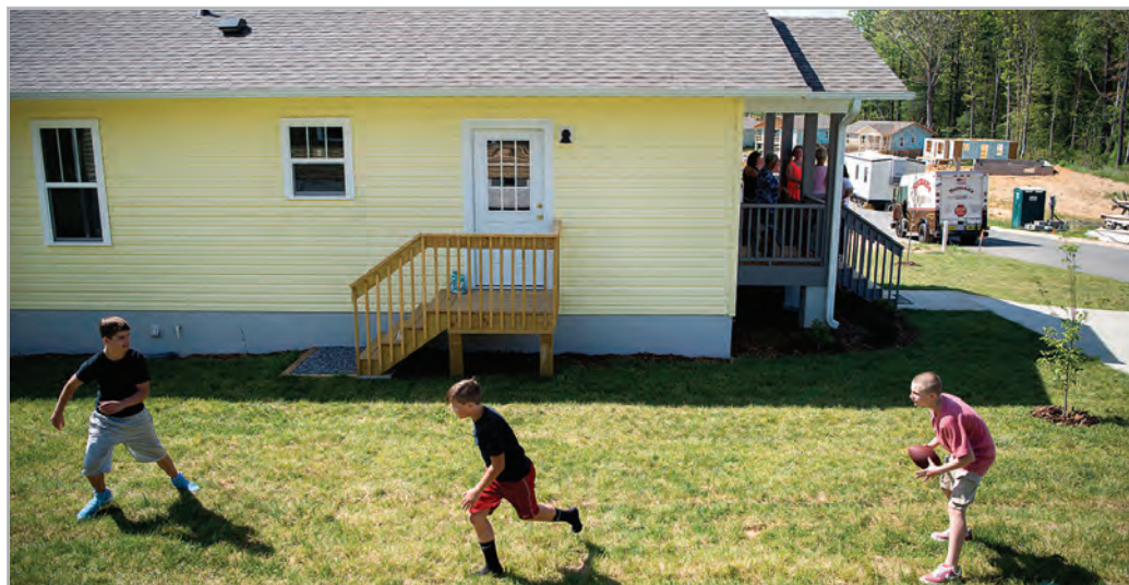
Children play football beside a Green Built Home in Asheville Area Habitat for Humanity's 21-house neighborhood being developed off of Beale Road in Arden. ASHEVILLE AREA HABITAT FOR HUMANITY PHOTO
