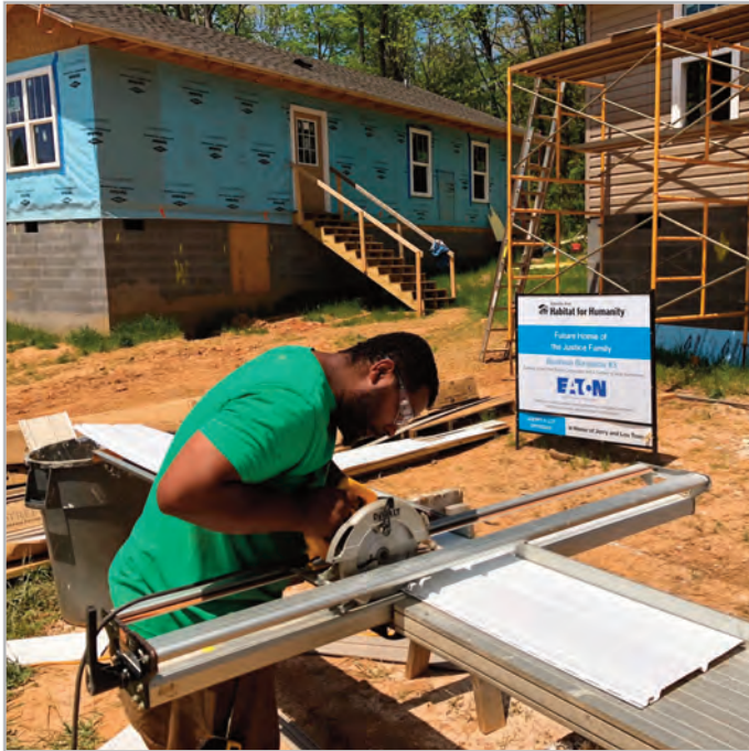
YouthBuild student Eddie Green volunteers on a Habitat for Humanity build site. He learned to use a track saw to cut soffit for the Habitat house. KAREN GEORGE PHOTO
