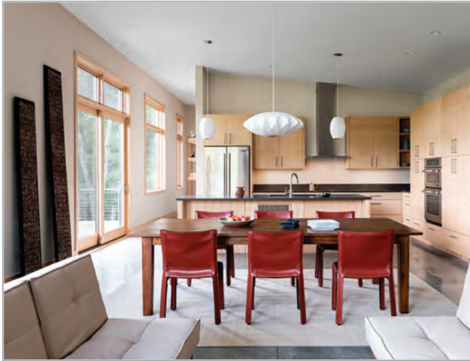
The polished concrete floor slab is sized to absorb solar heat gain in the day-time and release it into the home in the evening, passively heating the house.
