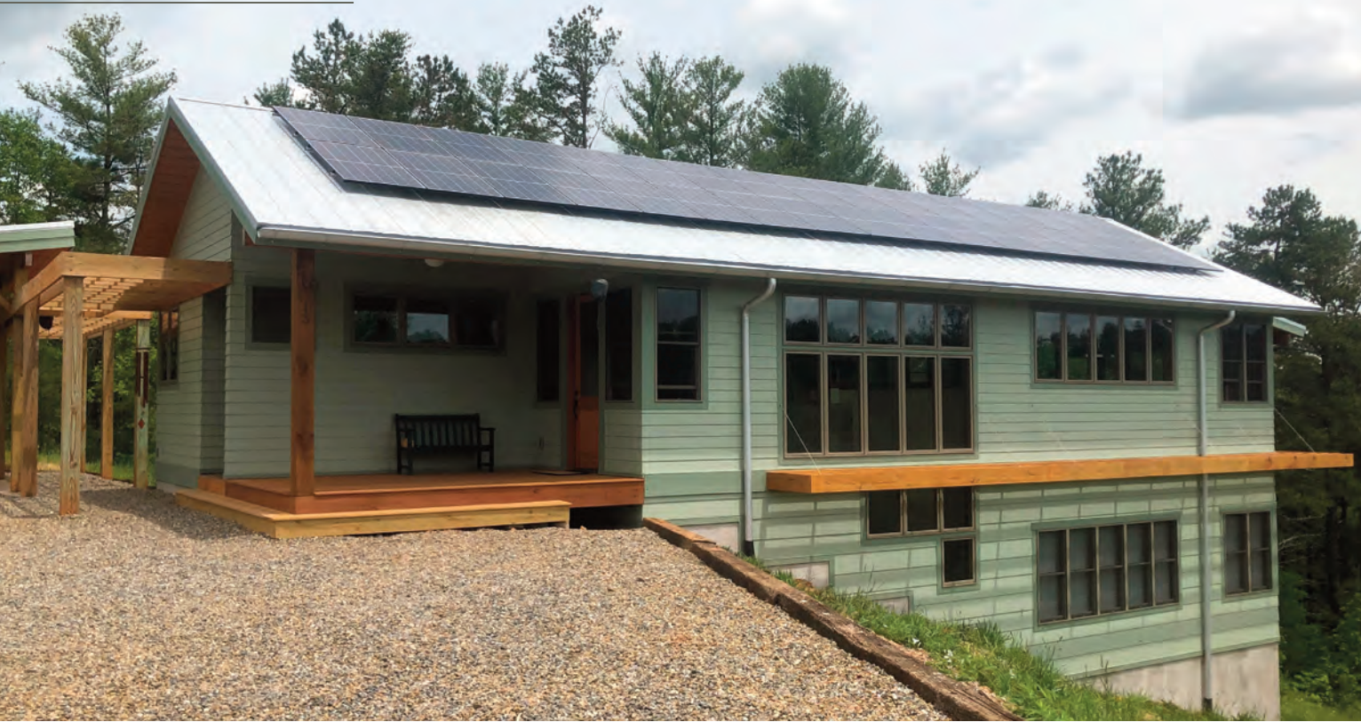
The 60-foot-long south side of the house is full of windows with high solar heat gain coefficient glass. MOUNTAIN SUN BUILDING & DESIGN PHOTOS
