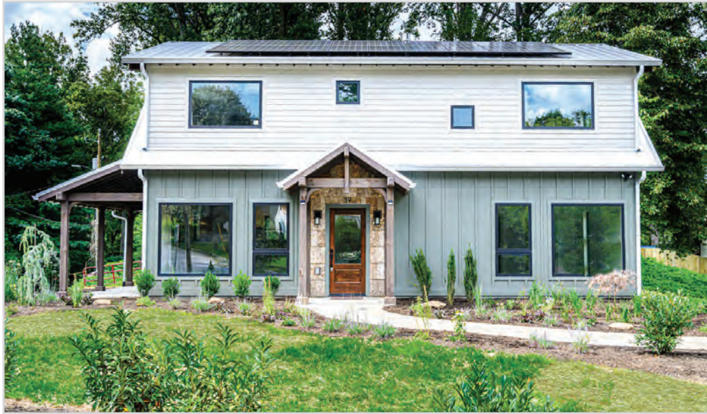
This Platinum Net Zero Energy Certified home was built by Familia Enterprises on an infill location in a walkable neighborhood. The home includes native and edible landscaping, and a variety of green finishes. FAMILIA ENTERPRISES PHOTO
