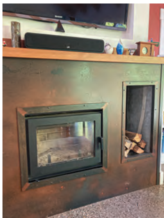
Amy Musser's personal wood-burning fireplace, built into a hearth. This fireplace has tightly closing gasketed doors and an outside air intake kit, and is EPA qualified and HUD approved for mobile home use.
