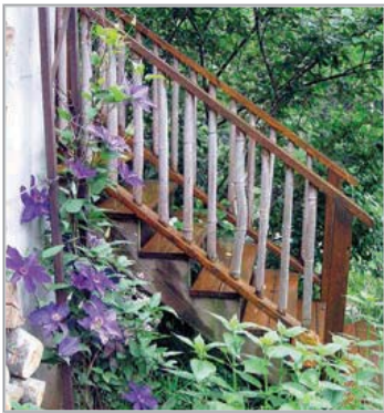
Bar top. (above) JAG Construction photo Bamboo balusters. Cady & Guyton Construction photo
