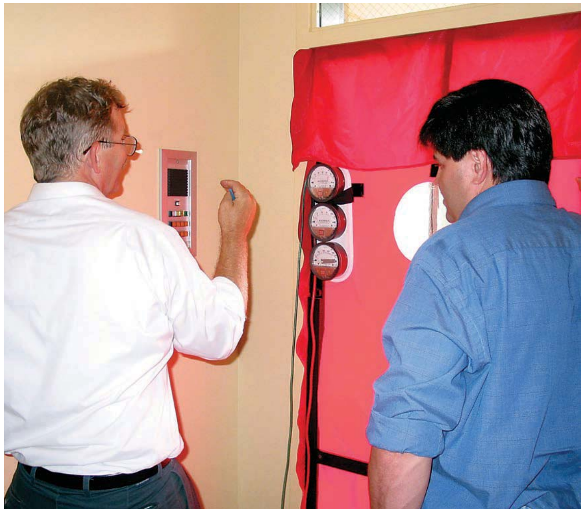
Conducting a blower-door test is essential to creating an airtight living space. Duncan Mcpherson, Samsel Architects photo
