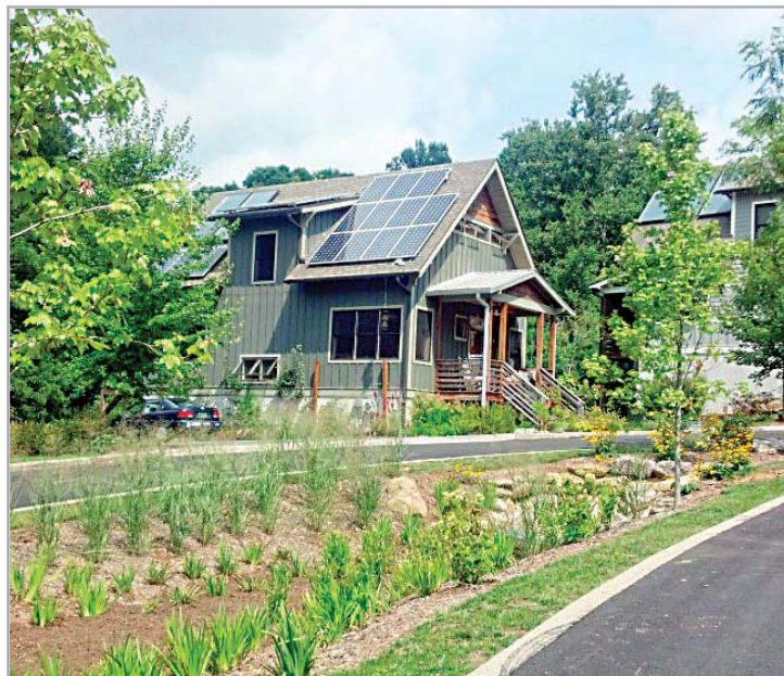
A low impact development and infill project, Davenport Park is located in west Asheville. Equinox Environmental photos
