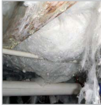
Completely blocked bath fan. (above) Saturated insulation and excessive mold. The owner found this after the tenant reported being sick. The water heater failed and flooded the crawlspace. The issue existed for two months before anyone found out. (right)
