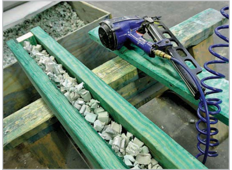
(left) A typical new construction can produce four pounds of waste per square foot. Green building aims both to reduce how much waste is produced and to divert excess material from the landfill. (right) We devised a method of insulating our headers by filling them with chipped up scraps of leftover polystyrene insulation board. Leigha Dickens photos
