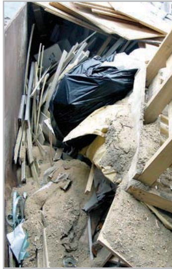
(left) A typical new construction can produce four pounds of waste per square foot. Green building aims both to reduce how much waste is produced and to divert excess material from the landfill. (right) We devised a method of insulating our headers by filling them with chipped up scraps of leftover polystyrene insulation board. Leigha Dickens photos
