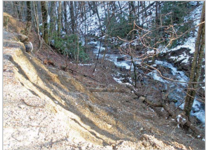
Left: Long Branch natural debris flow, Maggie Valley, Jan. 15-16, 2013. Above: Road embankment failure/debris flow, Maggie Valley, Jan. 15-16, 2013. Photos by Appalachian Landslide Consultants, PLLC
