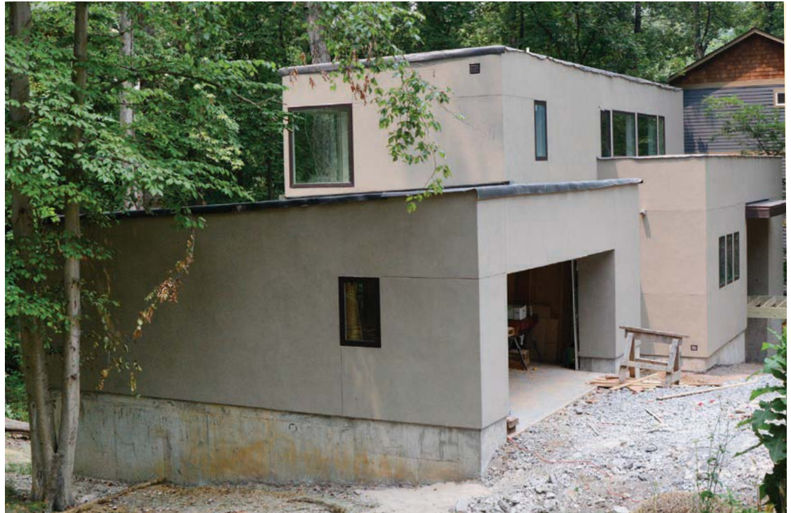
Located near Biltmore Village, this residential home utilizes green materials, with the key to the structure being structural insulated panels (SIPs). Bob Callahan (below). Garret K. Woodward photos
