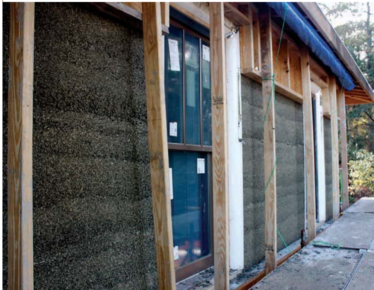
Hempcrete installation. Alembic Studio, LLC photo
