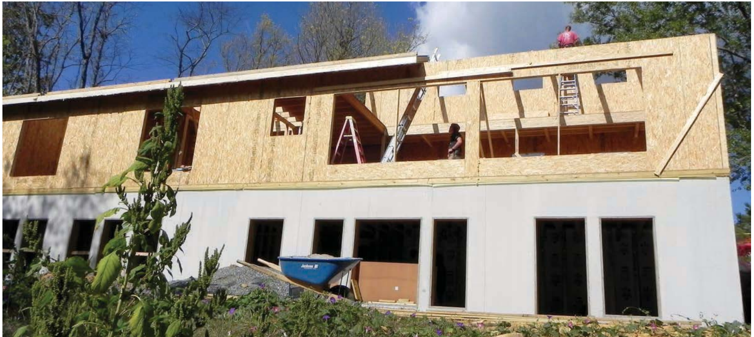
Structural insulated panels (SIPs) on a Superior Wall foundation for a passive solar home. VandeMusser Design photo
