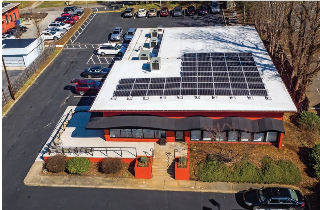
Asheville Yoga Center's 29.1 KW solar system by Sundance Power. Elliot Dunwoody photo
