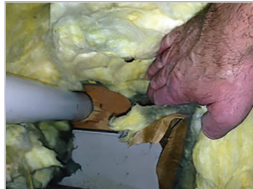
Above: Holes in the ceiling can waste a lot of energy. Here interior walls are drawing in hot attic air. Attic air sealing will stop this. Below, left: A blower door is set up for a Green Gauge assessment. Air leakage will be tested. Below, right: Interior wall top plates and plumbing holes as seen from the attic. These gaps allow a lot of air to escape or enter the home. Kevin Bauguss photos
